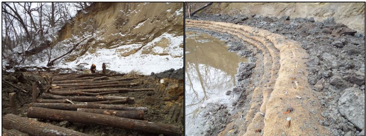
Figure 21. Toe wood and soil lifts, with seeding and woody cuttings, installed within Ravine Park, Sioux City Iowa (HR Green); an example of a much more volatile channel.
